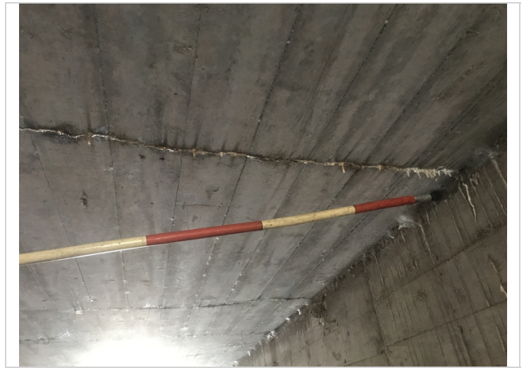
Barrel 1 has cracks with efflorescence in top of barrel. Common barrel 2.
