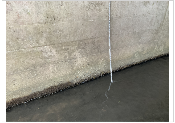
Barrel 1: Both barrels with abrasion at the bottom of the divider walls.
