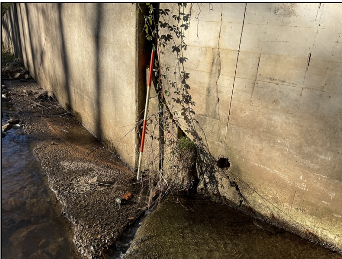
Outlet end barrel 1: Spall with exposed rebar.
