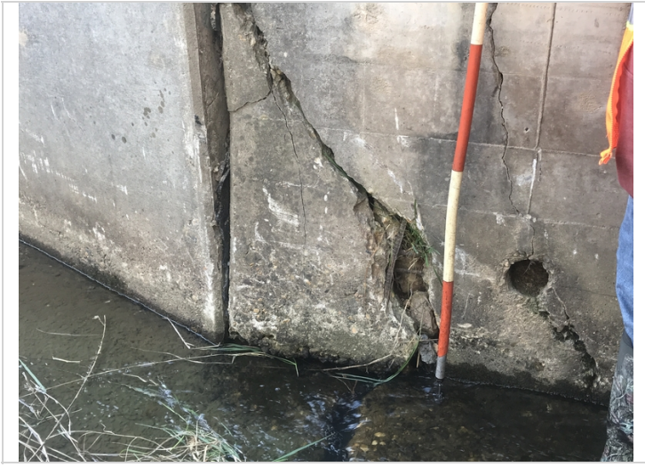
Outlet end of barrel 2 has exposed rebar.
