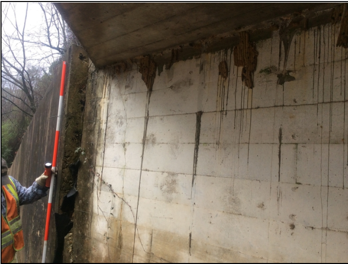
Wing wall at barrel 1 is leaning in due to scour action.
