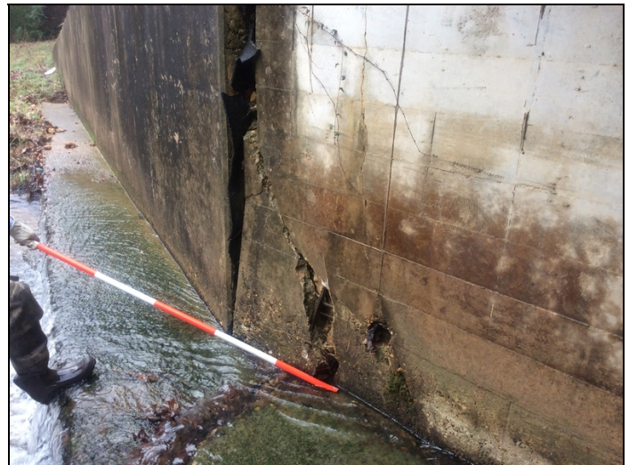
Barrel 1 outlet end spall with exposed rebar.
